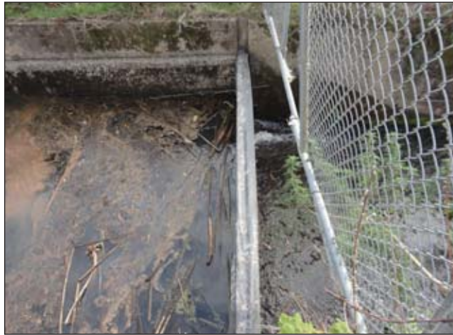
PHOTO 16: Denniston Dam spillway.
