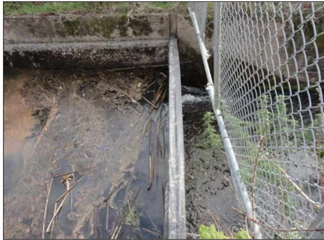
PHOTO 17: Denniston Dam spillway.
