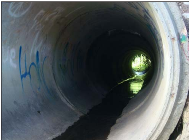
PHOTO 33: Existing barrier along Denniston Creek.
