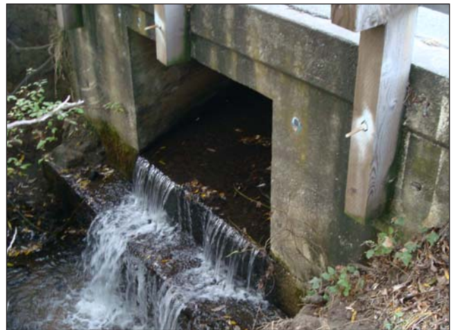
PHOTO 32: Existing barrier along Denniston Creek.
