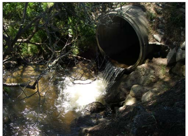
PHOTO 20: Existing barrier on Denniston Creek.
