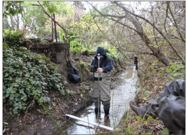
PHOTO 18: Downstream of Denniston Dam spillway.
