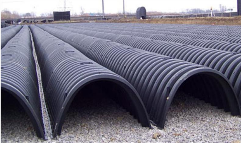
Figure 5.1. Installation of subsurface storage for a Regional Project. (Source: Conteches.com)
