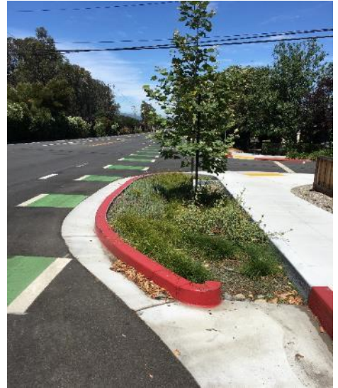
Figure 1.7. Stormwater curb extension, Carolan Ave, Burlingame. (Source: SMCWPPP)
