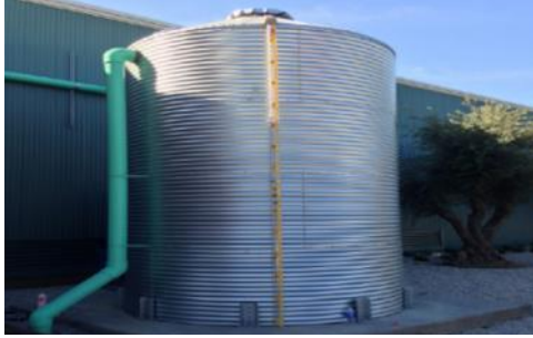
Figure 1.14. Rainwater harvesting cistern, Environmental Innovation Center, San José. (Source: City of San Jose)
