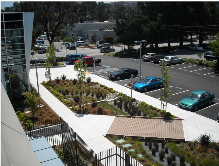
Figure 5.2. LID Retrofit Project in San Mateo County – Bioretention Area at Brisbane City Hall. (Source: SMCWPPP)
