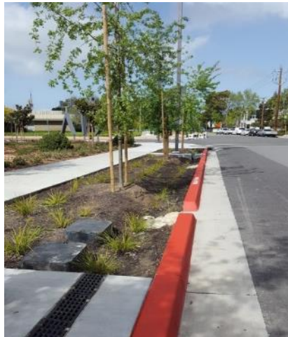
Figure 1.8. Stormwater planter, Hotel Nia, Menlo Park. (Source: City of Menlo Park)
